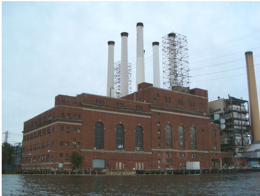
Glenwood Landing Power Plant with transmission lines threaded through structures at the top of the brick building (photo by Carol DiPaolo, 9/22/09)
