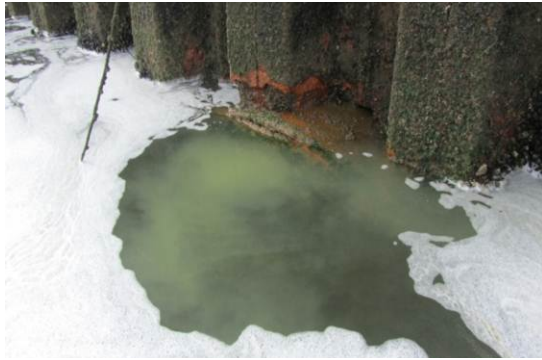
White flow from pipe at CSHH #10, Glen Cove Creek (photo by Carol DiPaolo, 6/8/11)
